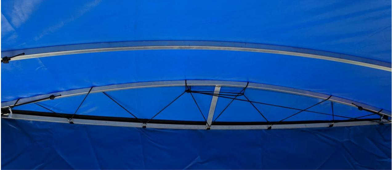
Tie the rope to the farthest end ring in one of the corners. Make sure the rings are routed under the end bow of the canopy and hang slightly below the end bow. Begin to thread the rope under the end bow. Then route the rope under the first mid bow and then up and over it. Continue pulling the rope through and into the next ring. Repeat this step until you have threaded the rope through all of the end rings.
